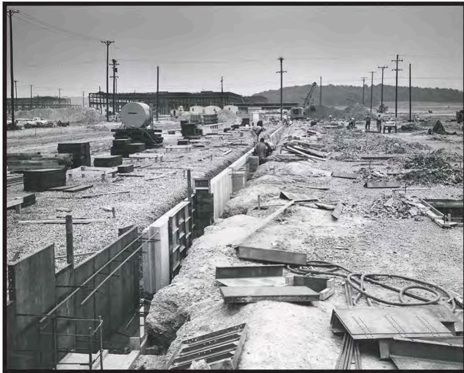
Figure 8: Foundation Work for the X-326 Process Building, October 1953
